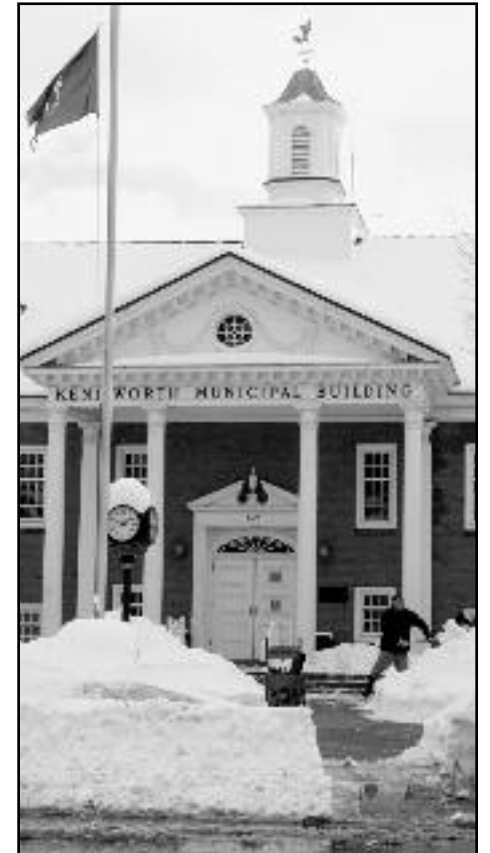
(above, l-r) DPW workers cleaning up the Municipal Building.
