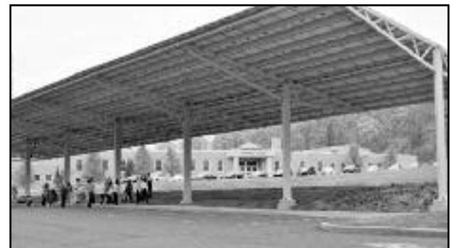
(above) New solar panel array at Bayberry School.
