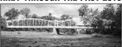
(above) New to the tour this year is the Elm Street Bridge, Elm Street (CR 667) at intersection with River Road (CR 567) between Hillsborough & Branchburg Townships. The Elm Street Bridge, one of the last remaining of its type in the State, consists of two (2) single span lenticular through trusses over the South Branch of the Raritan River between Branchburg and Hillsborough Townships. The bridge was constructed in 1896, stiffened in 1932 and rehabilitated for continued vehicular use in 1984.
