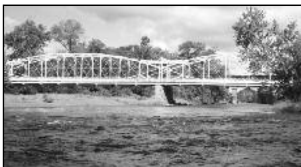
(left) New to the tour this year is the Elm Street Bridge, Elm Street at intersection with River Road between Hillsborough & Branchburg Townships. The Elm Street Bridge, one of the last remaining of its type in the State, consists of two (2) single span lenticular through trusses over the South Branch of the Raritan River between Branchburg and Hillsborough Townships.
