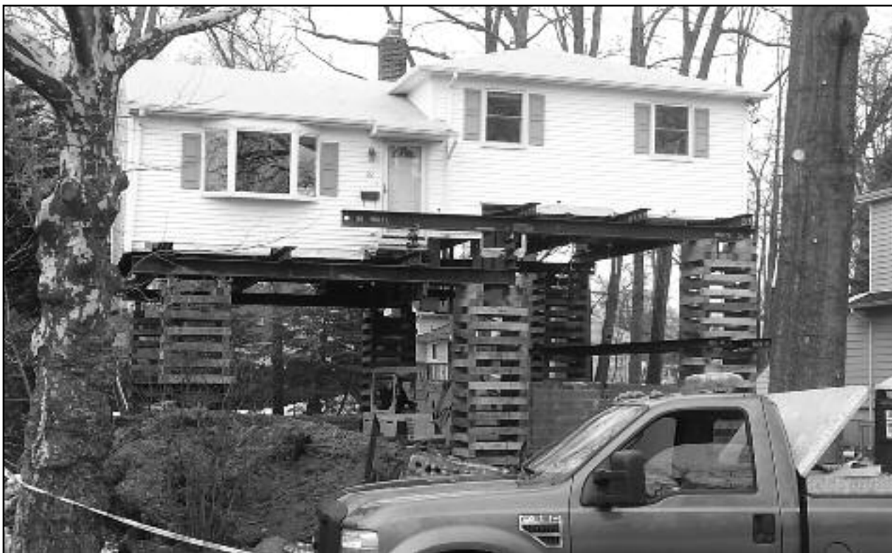
(above) This house, located in Cranford on Riverside Drive across from the river and the dike, is one of several in town being elevated to protect it from flooding. The house will have an approximate 12 ft cement wall supporting it.
