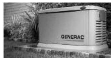
Automatic Standby Generator
