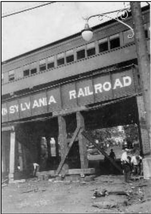
(above, l-r) Two photos from a roll of film that Hector Conforti shot of a train accident where passenger cars derailed and fell from the elevated tracks. The trestle over South Street had to be braced during the months-long repair.
