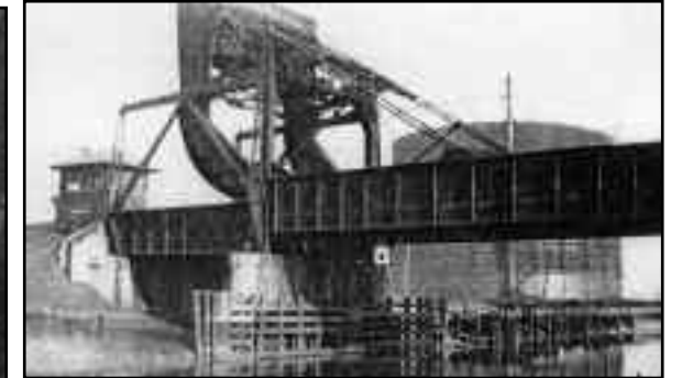
Railroad Bridge over Crick next to Gas House.
